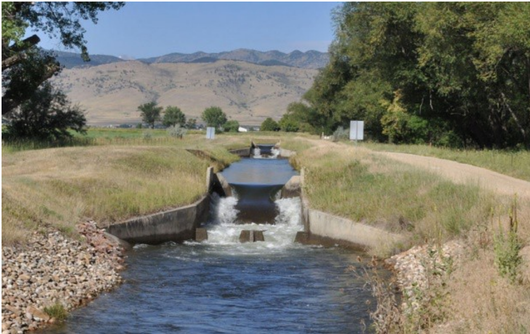
Figure 2 An example of a typical drop structure: a drop structure on the Boulder Feeder Canal, sourced from NorthernWater.org.
