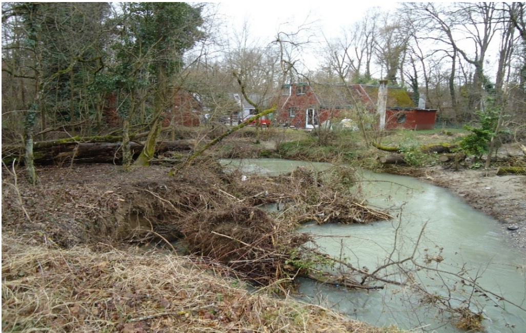
Figure 5 Eroded bank at around 4km upstream of the D/S end (Photo taken on 4.03.2014).
